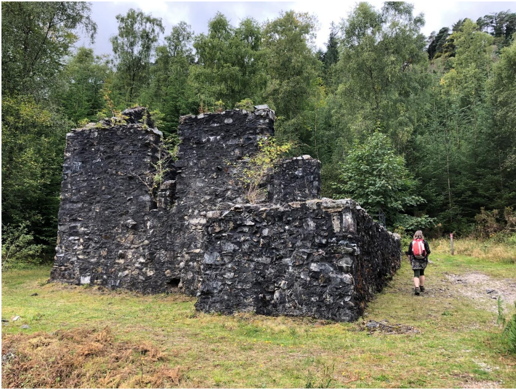
Some of the abandoned mine buildings in the Gwydyr Forest.
